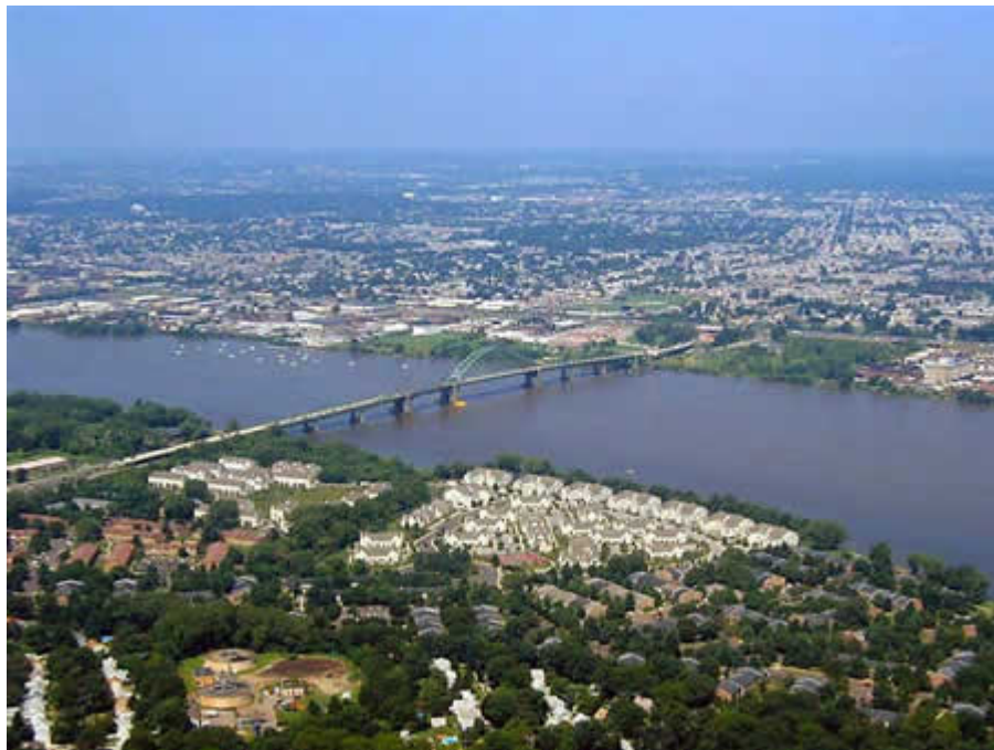
The Talcony-Palmyra Bridge-Looking Southwest
